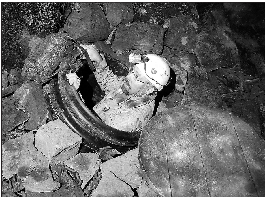
Figure 3. Dug entrances may be stabilized using culvert pipe. A lid may be fitted to control air flow and temperature fluctuations. In most cases, the management objective at the new entrance will be to maintain the cave in the same condition as before the new entrance was opened. In this example surface disturbance and visual impact are minimal. Photo by P.C. Lucas.
