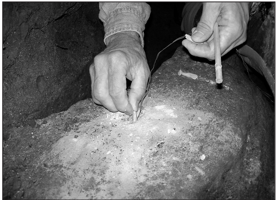
Figure 1. Rock shaving techniques using soda straws filled with pistol powder and inserted into a drilled hole in the rock create a very controlled splitting or shaving of the rock without the potential damage associated with more traditional explosives. Photo by W.K. Jones
